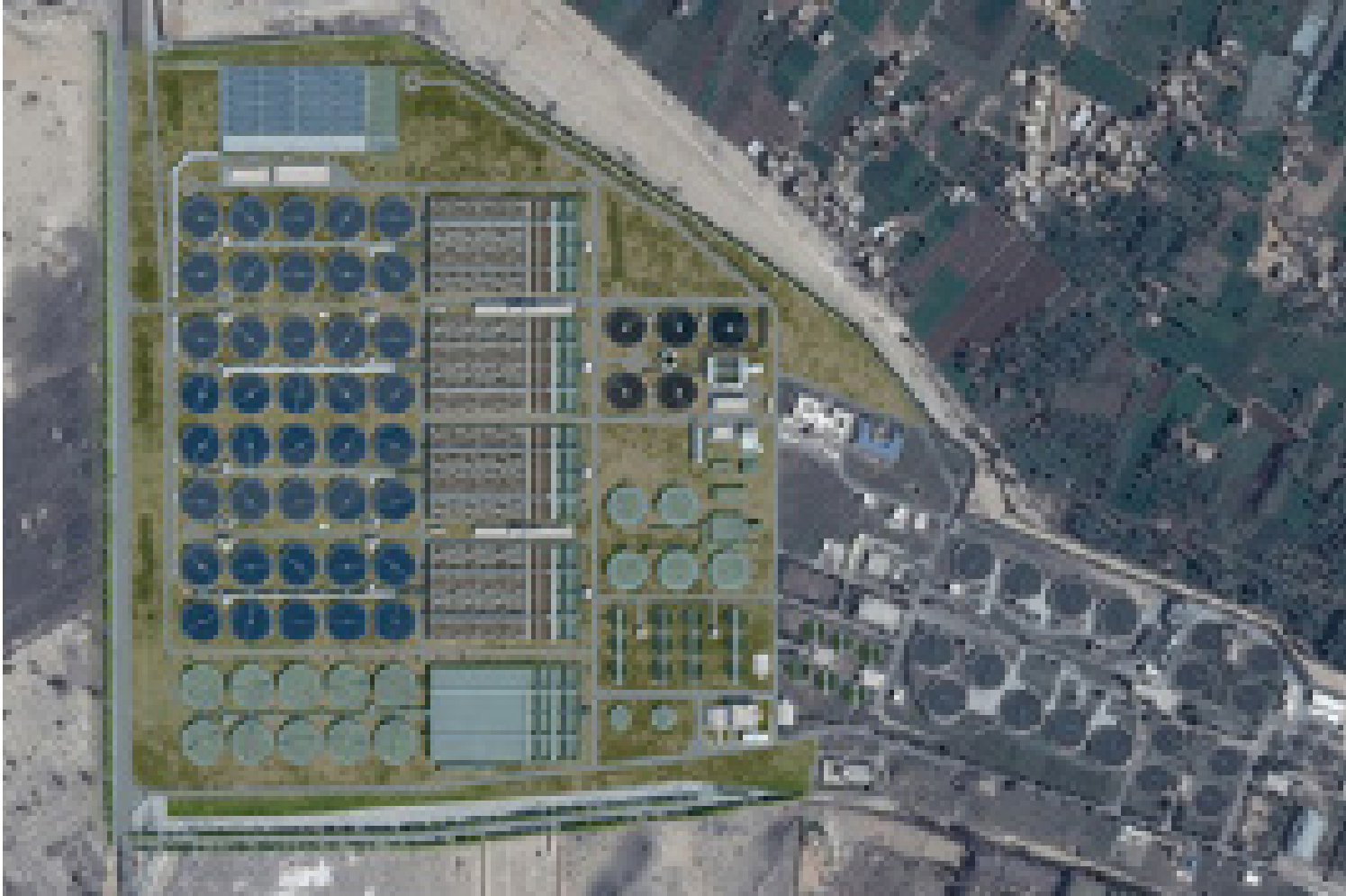
Aerial view of the current wastewater treatment plant.
